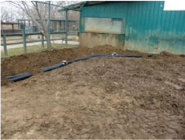
Drain lines are laid and then tons of fill dirt are brought in to raise up the soil level.
