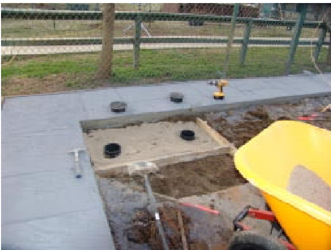
Concrete walkways poured around the perimeter of the enclosure will not cause water to back up inside the habitat because there are underground drain lines that lead rainwater away.
