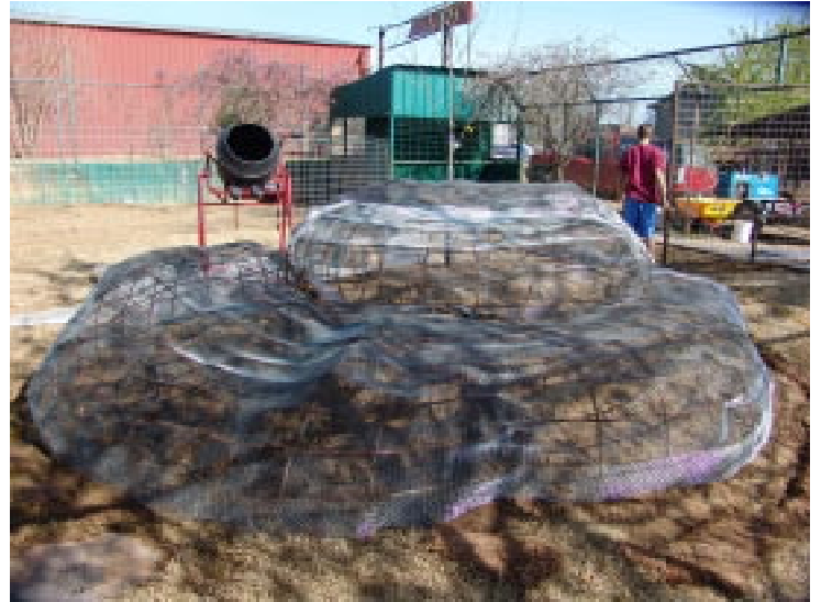
An artificial boulder is fabricated out of rebar and expanded metal lathe, then covered with a mix of Portland cement and vermicu-
