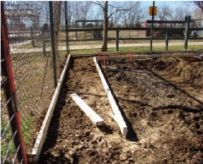
Wooden forms are erected in preparation to pour concrete walkways around the perimeter.
