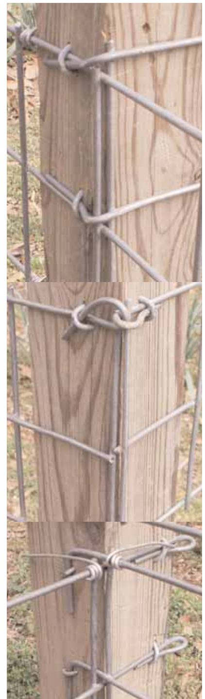
Top to bottom: (top) Joinery with one panel inside, one panel outside. Cage is to right.
