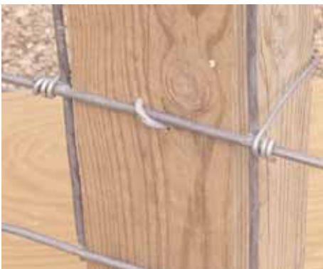
Joining to a line post
