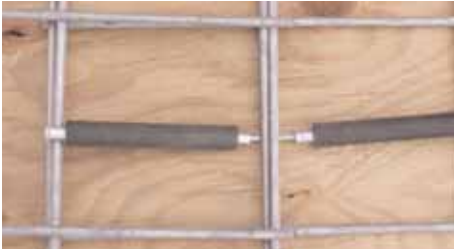
Use of wire wrapping tools to join panels.
