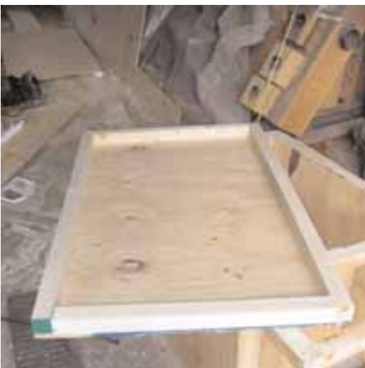
The floor is a simple 2 x 2 frame covered in plywood and...
