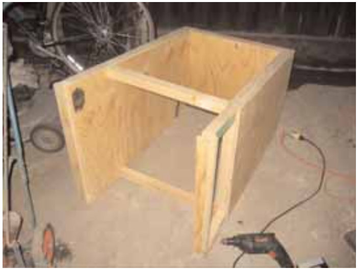
Sides are attached to the back wall. Slider rails for front baffle are attached to front edge of side walls.
