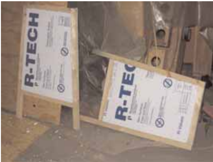
Left and right side frames with polystyrene insulation in place.
