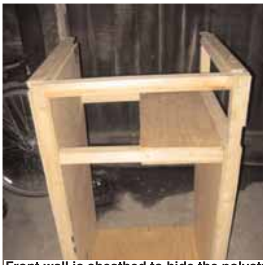
Front wall is sheathed to hide the polystyrene. Bottom stop for the baffle is installed at the lower end of the baffle rails.
