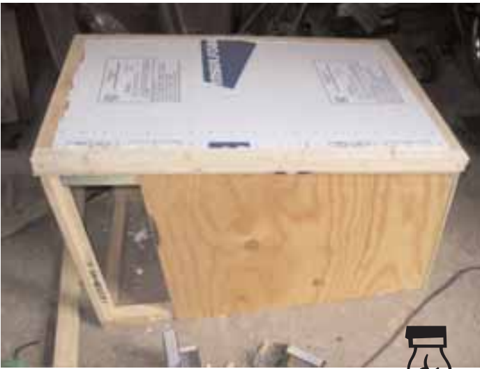
Roof likewise is filled with polystyrene.
