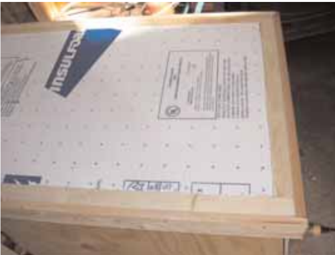
Detail showing how the 1 x 3 wood is attached outside the frame to eliminate drafts.
