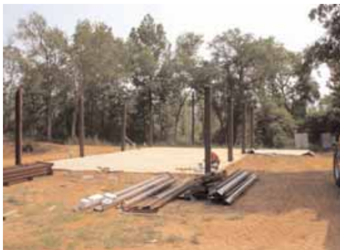
Concrete slab and first support poles.
