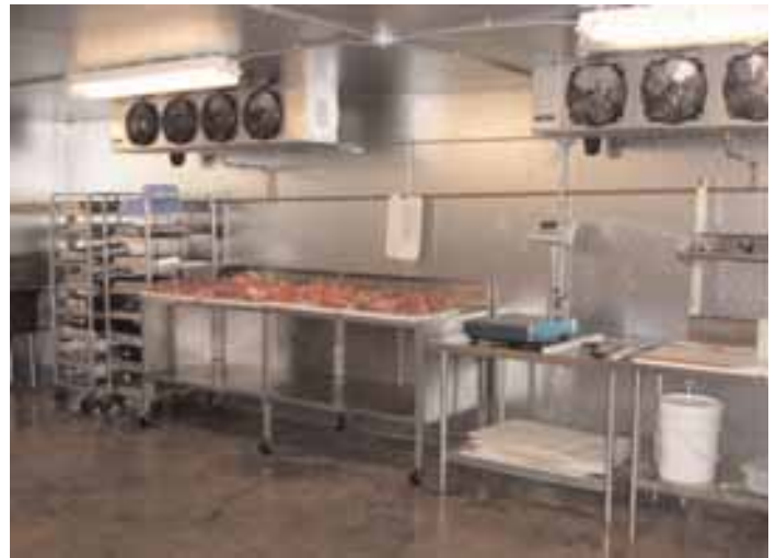
Food preparation area. Note refrigeration units and environmentally-sealed fluorescent lights.
