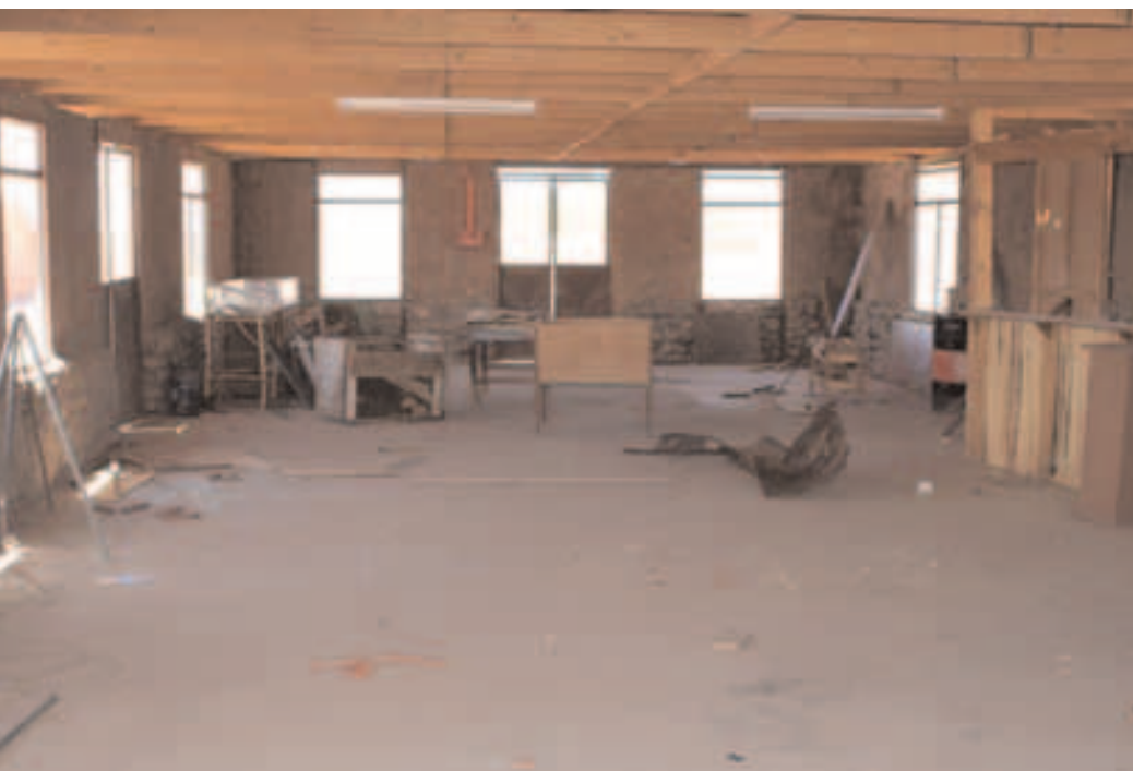
The interior of the building with exposed roof trusses. The roof is open on the sides and not insulated. There is no water to the building.
