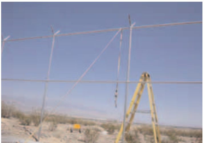
21. Mike is attaching top rail sleeve to the top rail, following the string attached to poles, which is used as a guide to make sure all is in a straight line
