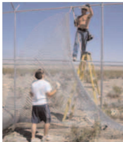
23. Fellow FCF member Brian Ferko is attaching the tension bar to the 6 gauge chain link fabric. Tension bar can also be attached after the fabric is already hanging from the frame. Fabric should be attached to the frame from the inside.
