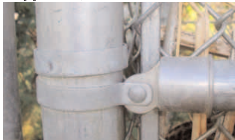
13. Line rail clamps are used to attach middle and bottom rails to the regular line posts. Fence wire ties are used to attach chain link fabric to the rails and posts.
