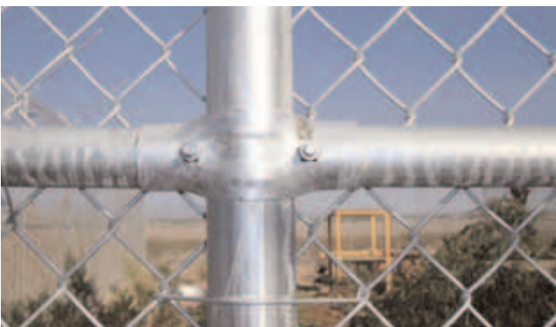
14. Picture shows the use of tension bands to attach the chain link to the posts and to the door frame. It also demonstrates the attachment of the middle rail and above the door rail to the gate posts using rail end and rail end band.
