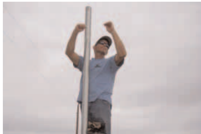
20. Scott and Mike keep working on the cage frame, attaching the top rail to the posts, through the V-barbed wire arm.
