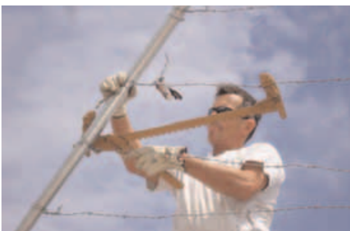
28. Finished the top of the cages with barbed wire attached, showing the use of corner V-barbed wire arms above the door. The short black sticks are the optional hot wire attachments.
