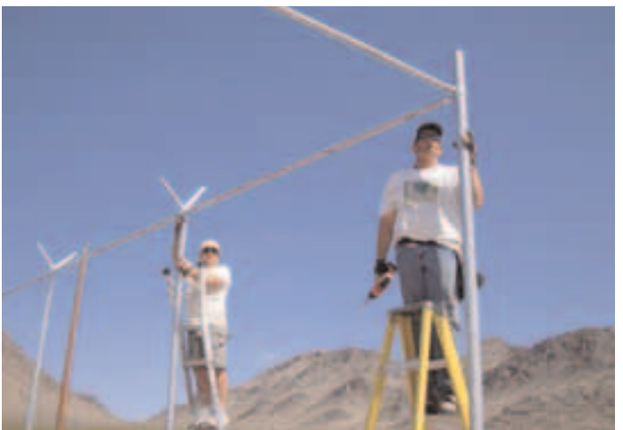
21. Mike is attaching top rail sleeve to the top rail, following the string attached to poles, which is used as a guide to make sure all is in a straight line
