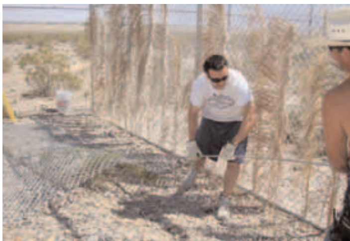
24. Brian and Scott attaching 6 gauge chain link with the help of tie down straps and winch or rope.
