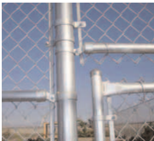
15. Top rail sleeve is used to attach two top rails
