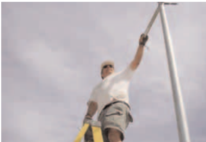
22. Once the cage frame was finished, with all the poles and top, middle and bottom rails in place, it was time to hang the chain link, using ladders and different tie downs and winch straps to get it up to the 12 foot height.
