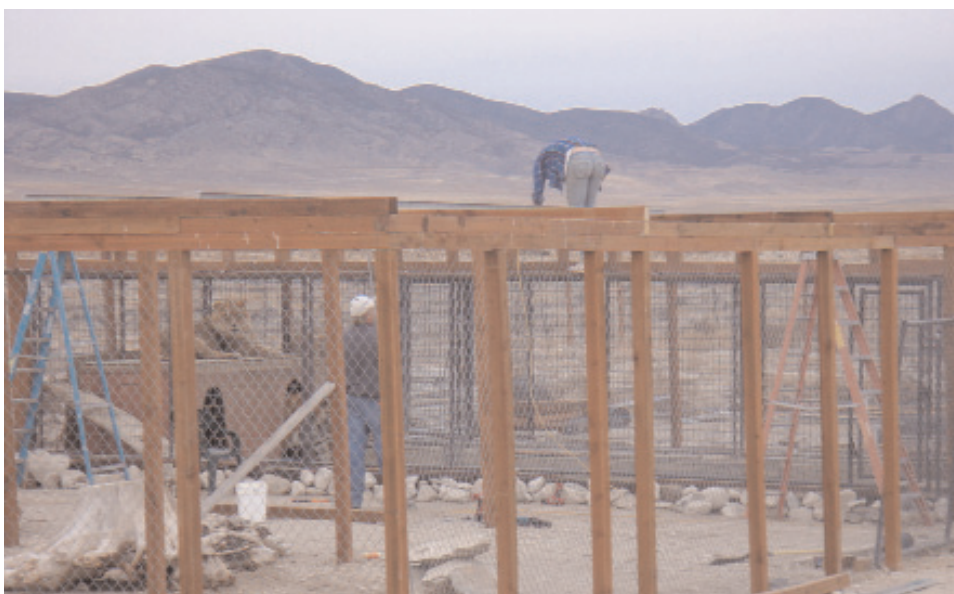
Once we decided to roof over the original cage, we had to cut down the recurve and some of the wall height. Deanna Croasmun
