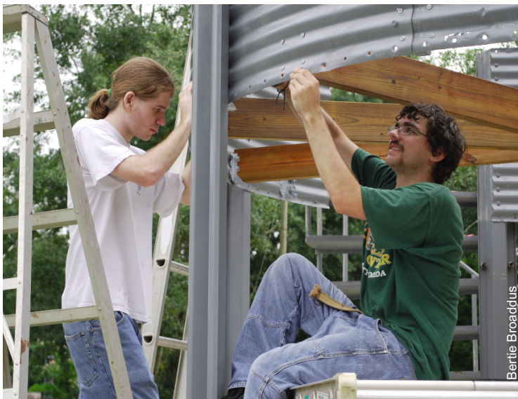
Bear Creek interns work on the Center's latest project, a tall observation tower (made from a converted grain bin) that will overlook the new serval habitat, future home to a mixed group of these spotted African cats.
