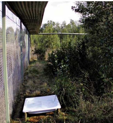
Fernando provides large, open areas for the guíñas, and keeps them confined with an ingenious use of horizontal, metal roofing that attaches to the top of the welded wire mesh walls.
