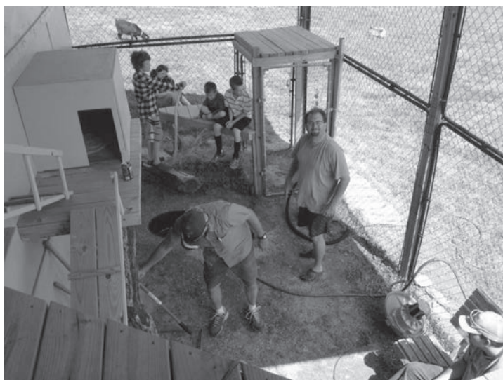
Everyone helped build Nyasha the serval, a big habitat that attaches to the kitchen.
