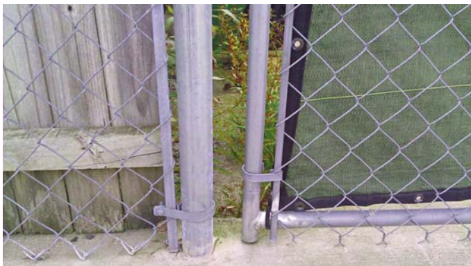
Large gap between the gate pole and the pole where the gate latches to the pole leave room for unwelcome visitors.
