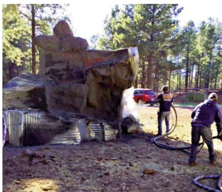
At Bearzonia, large natural-looking rock formations are sculpted out of scrap metal and cement.
