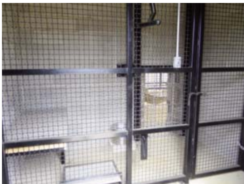
Woven mesh for indoor housing/feed area. Square tubing for gates.
