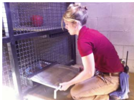
After tray is put inside feed slot, lid is then pulled out and placed vertically. The cat cannot reach the keeper.
