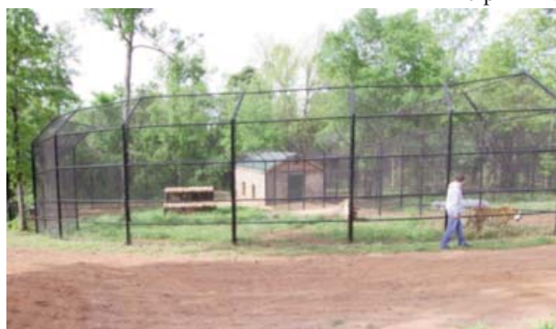
Tiger/Lion Enclosure is constructed of 12-foot vinyl-coated chain link with 4-foot recurve. Rub rail keeps chain link from bowing out when cats rub along the fence.
