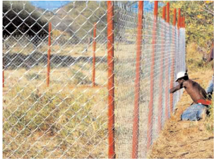
The latest boma design is a square rather than round enclosure, and uses metal instead of wooden posts.
