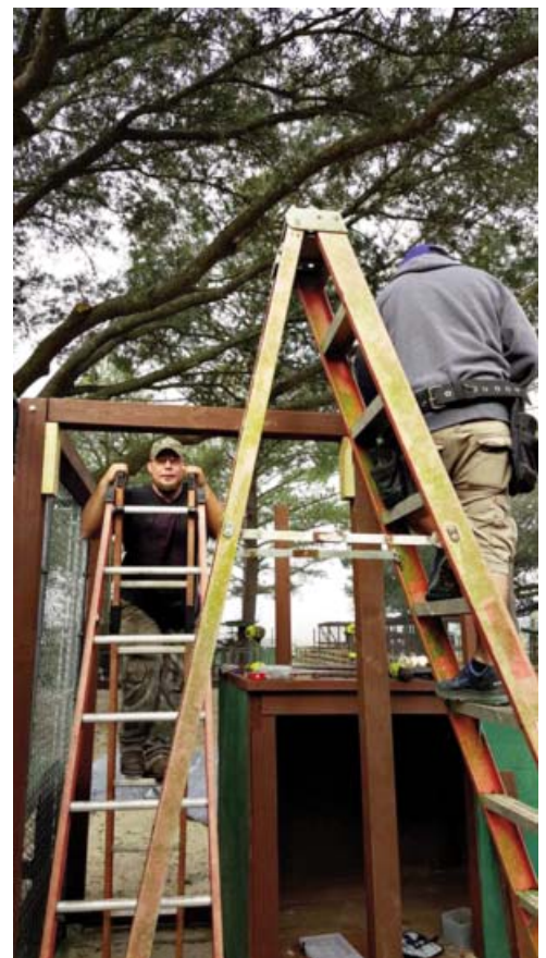
Volunteers James and Jeremiah building the 15-foot lockout extensions for Bo and Lepa.
