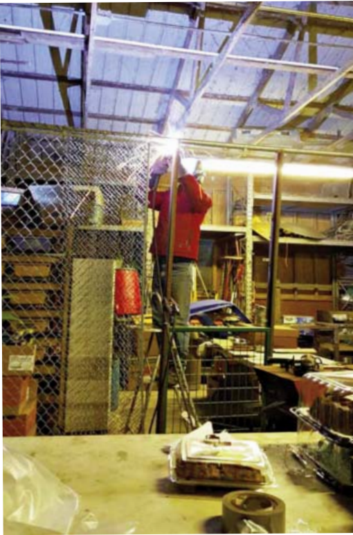
Robert Chaples welding guillotine doors in the new enclosures.
