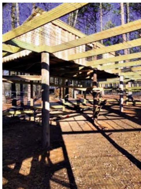
A creative attic area has holes all over to allow Gibs access into and out of the covered area.
